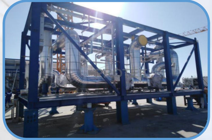
INSULATION FOR SKID MOUNTED PIPING – USA
