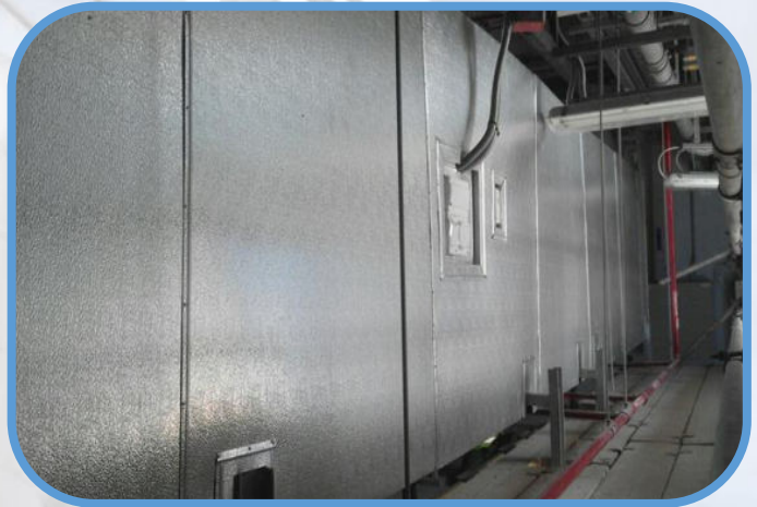
CLADDING FOR HVAC DUCTS – DWTC
