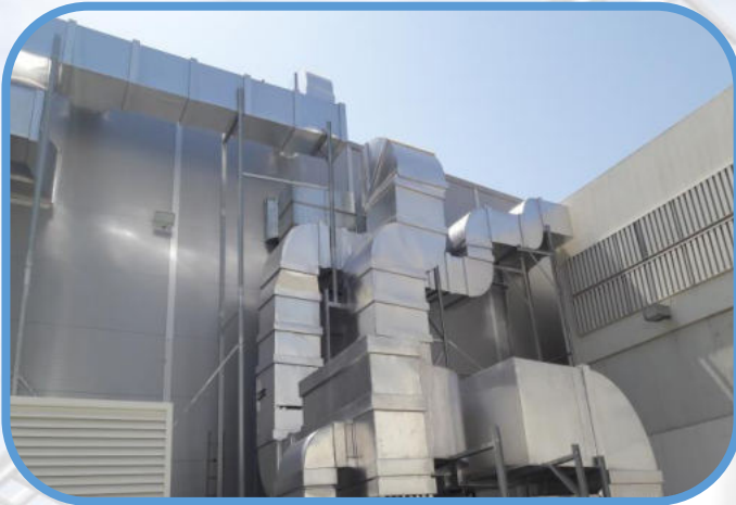
CLADDING FOR HVAC DUCTS – DWTC
