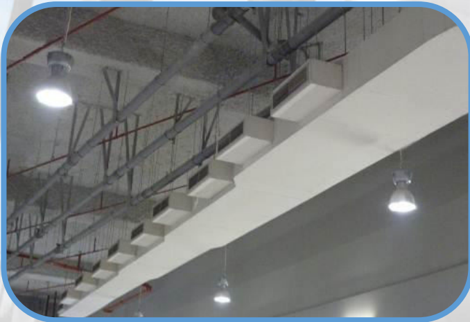
FIRE RATED ENCAPSULATION – RIHAN HEIGHTS, ABU
