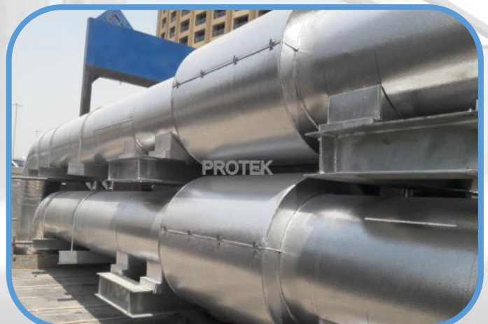
CLADDING FOR HVAC DUCTS – DUBAI MALL
