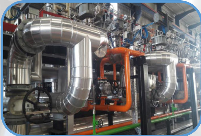
INSULATION FOR SKID MOUNTED PIPING – INDIA
