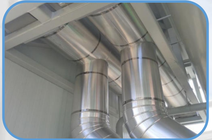
CHILLER UNIT INSULATION AND CLADDING -
