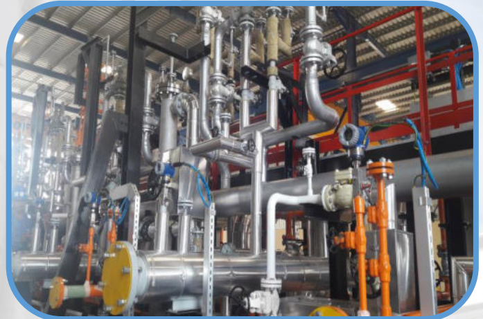
INSULATION FOR SKID MOUNTED PIPING – INDIA
