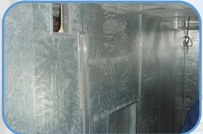
ACOUSTIC INSULATION FOR ENGINE ROOM
