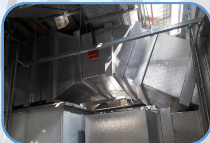
CLADDING FOR HVAC DUCTS – DUBAI MALL
