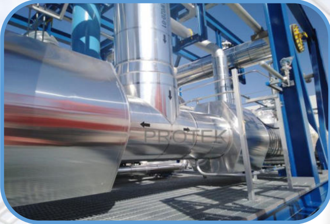
INSULATION FOR SKID MOUNTED PIPING – USA
