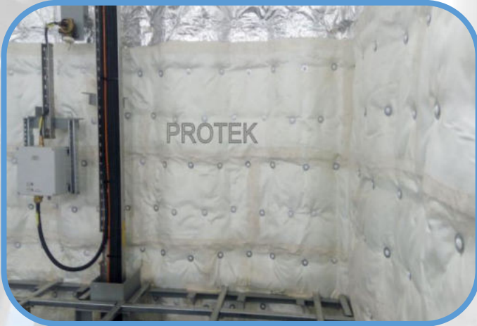
INSULATION FOR OFFSHORE PLATFORM
