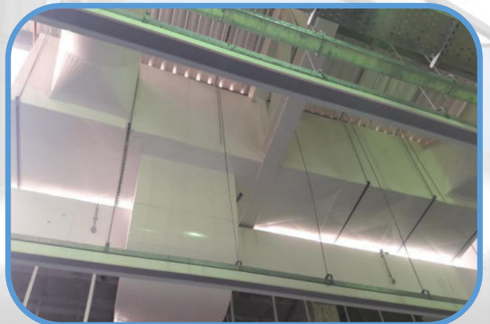
POWDER COATED SHEET CLADDING FOR HVAC
